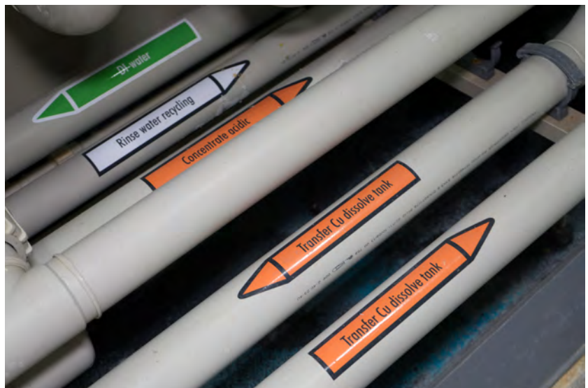
Figure 8: Atotech tank transfer plumbing automates chemistry change-over and maintenance.
