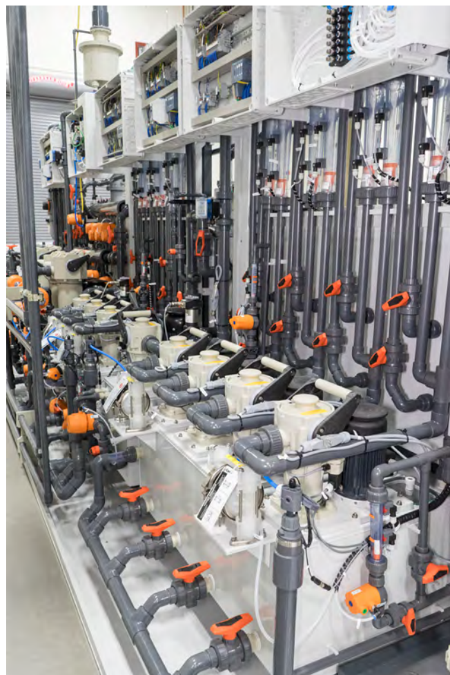
Figure 7: Plumbing, controls, and tanks provide AWP's chemistry and environmental controls.
