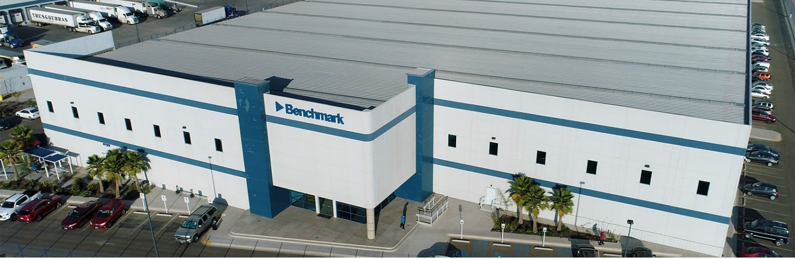
The facility in Tijuana, Mexico.
