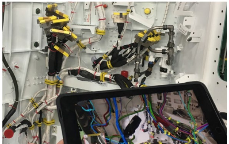
AR Applied to Harness Installations. (Source: Lockheed Martin Corp.)
